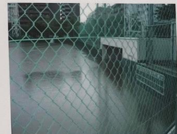
雨水貯留時 Storing stormwater
